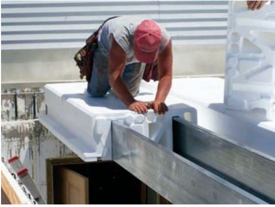
Stacking the AmDeck® Floor & Roof System.
