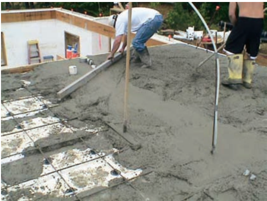
Smoothing concrete to create a flat surface.
