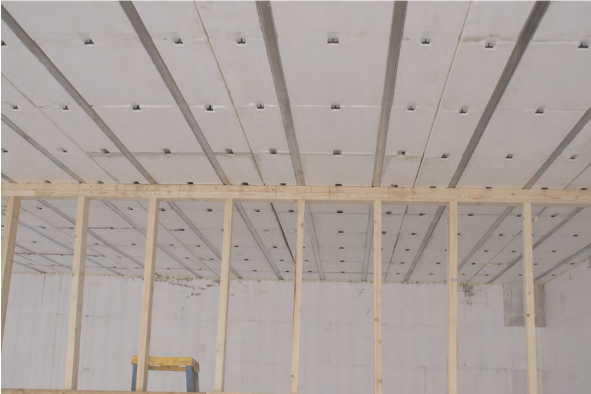
Figure 4.2 – Shoring beneath AmDeck™ floor
