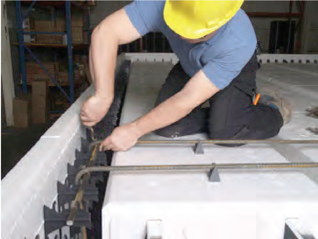
Figure 7.22 - Tying the top slab reinforcement with the horizontal bars on ICF wall
