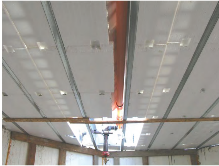
Figure 6.3 – Fire sprinkler system attached to steel joist
