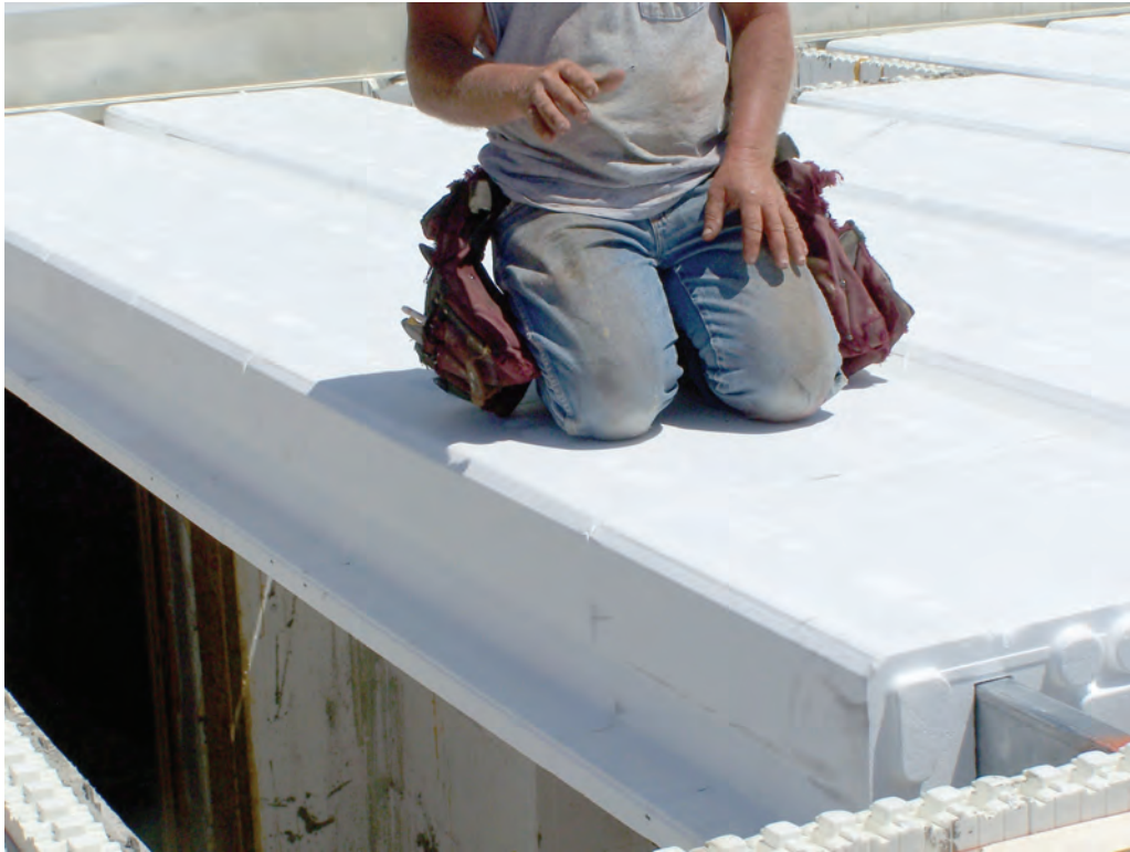
Figure 7.12 – A completed AmDeck™ row
