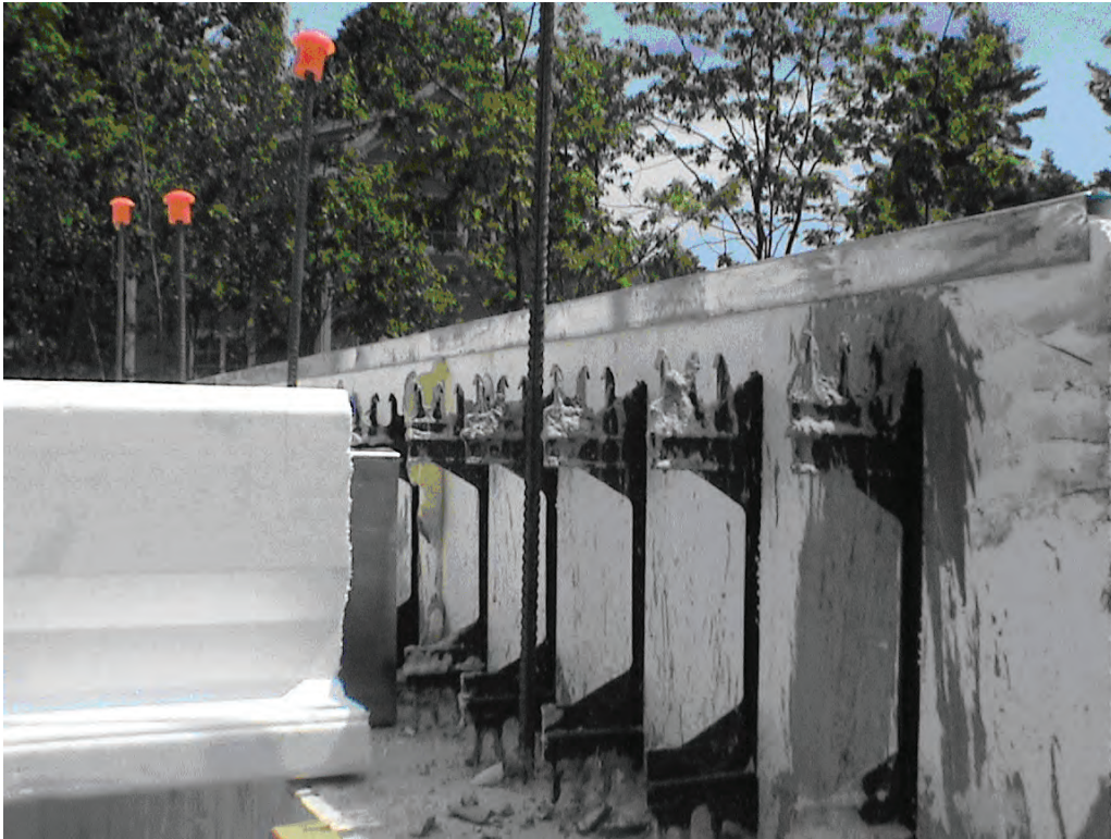
Figure 7.20 - Amvic ICF cut halfway
