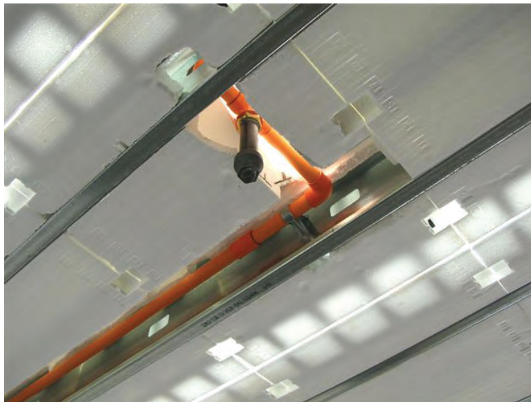
Figure 6.4 – Large pipe attached to steel joist
