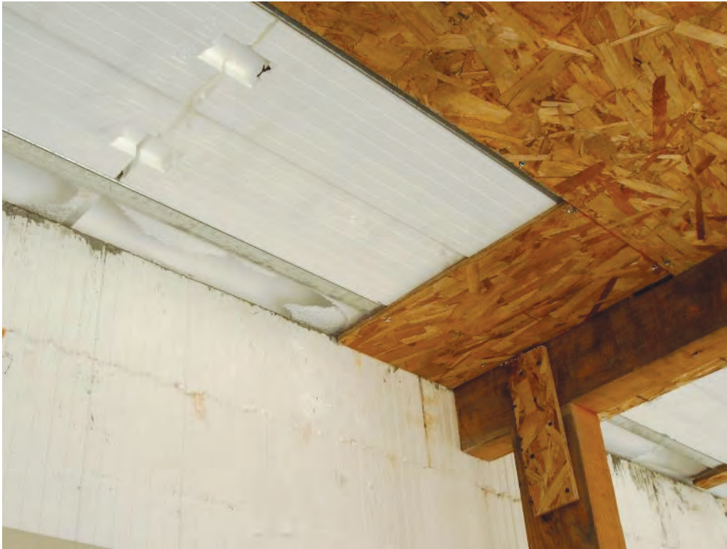
Figure 7.14 – Longitudinally cut AmDeck™ block, supported by OSB board
