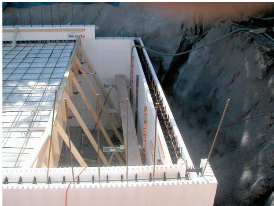
Figure 7.25 – Bracing the formwork for concrete beam
