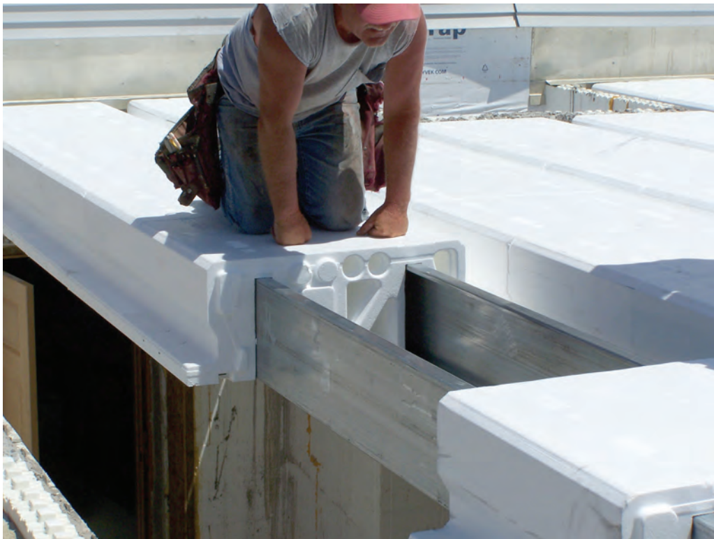
Figure 4.1 – Laying out forms
