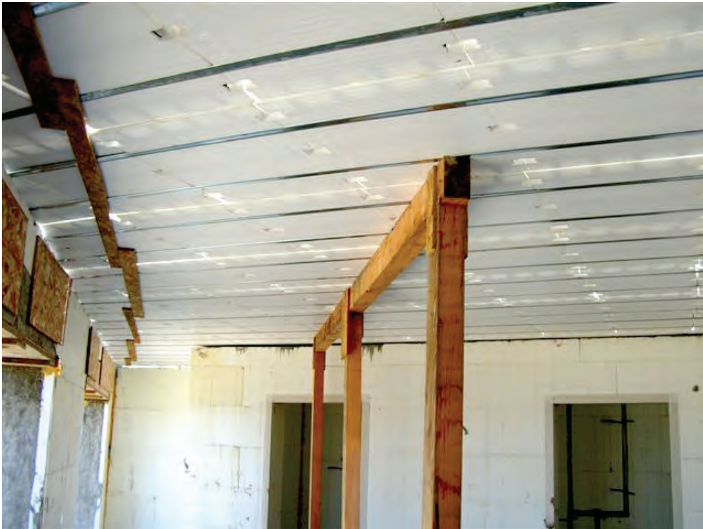
Figure 7.28 – Extra bracing for AmDeck™
