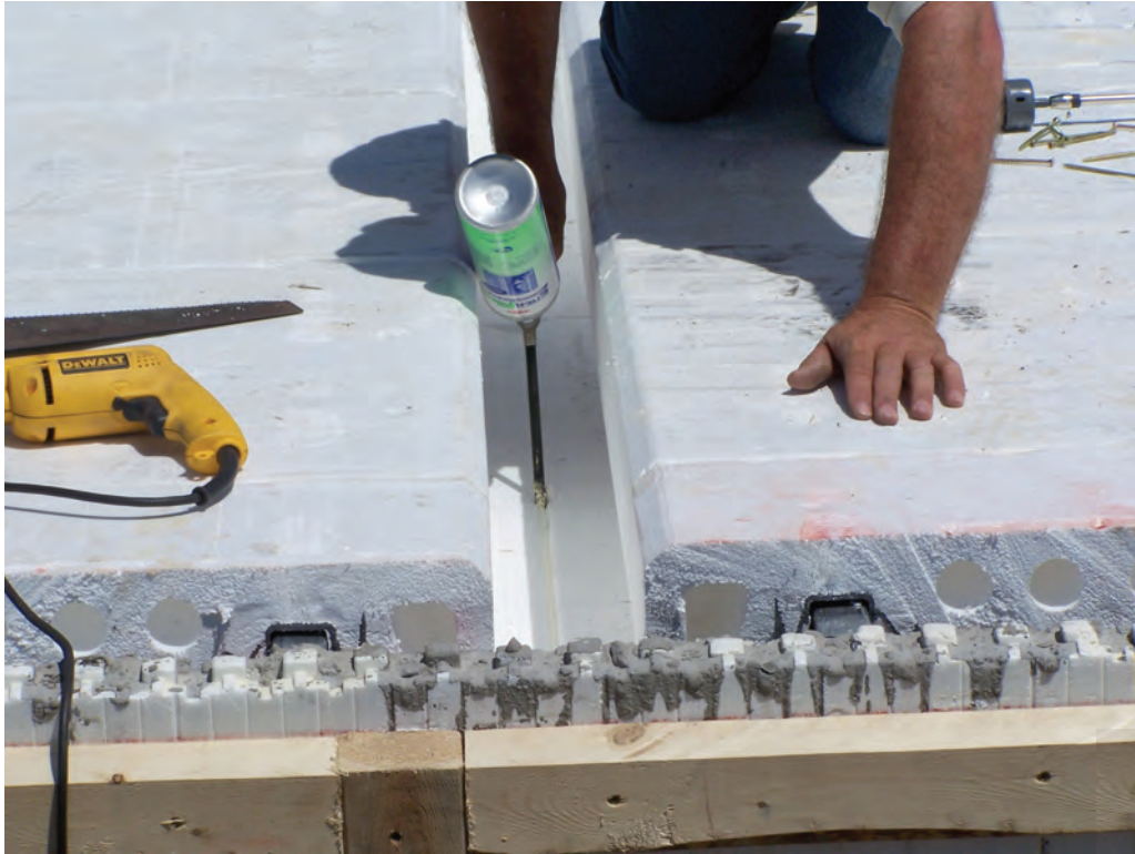
Figure 4.3 – Sealing seam between AmDeck™ blocks
