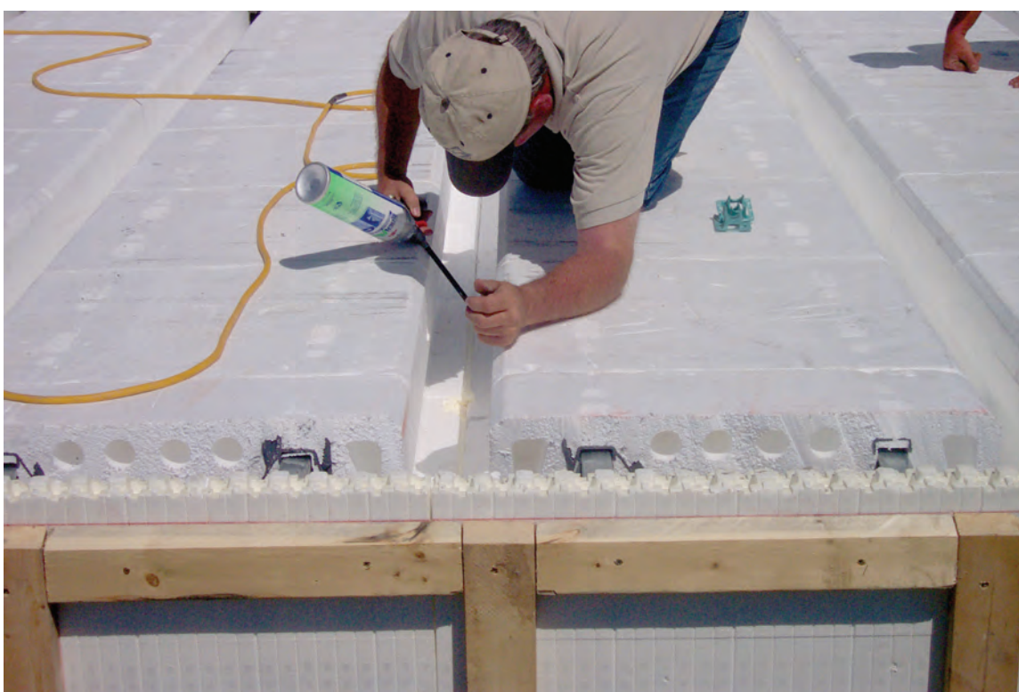
Figure 7.15 – Sealing gaps between AmDeck™ forms
