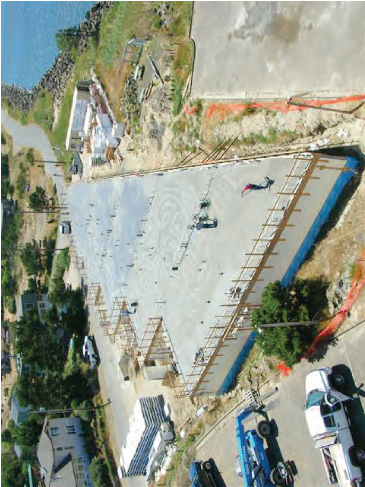
Figure 8.8 – Stage 2: Final Finishing of Concrete on AmDeck™
