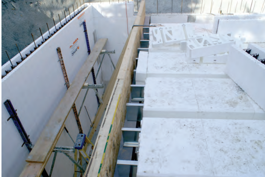
Figure 7.24 – Formwork for concrete beam construction
