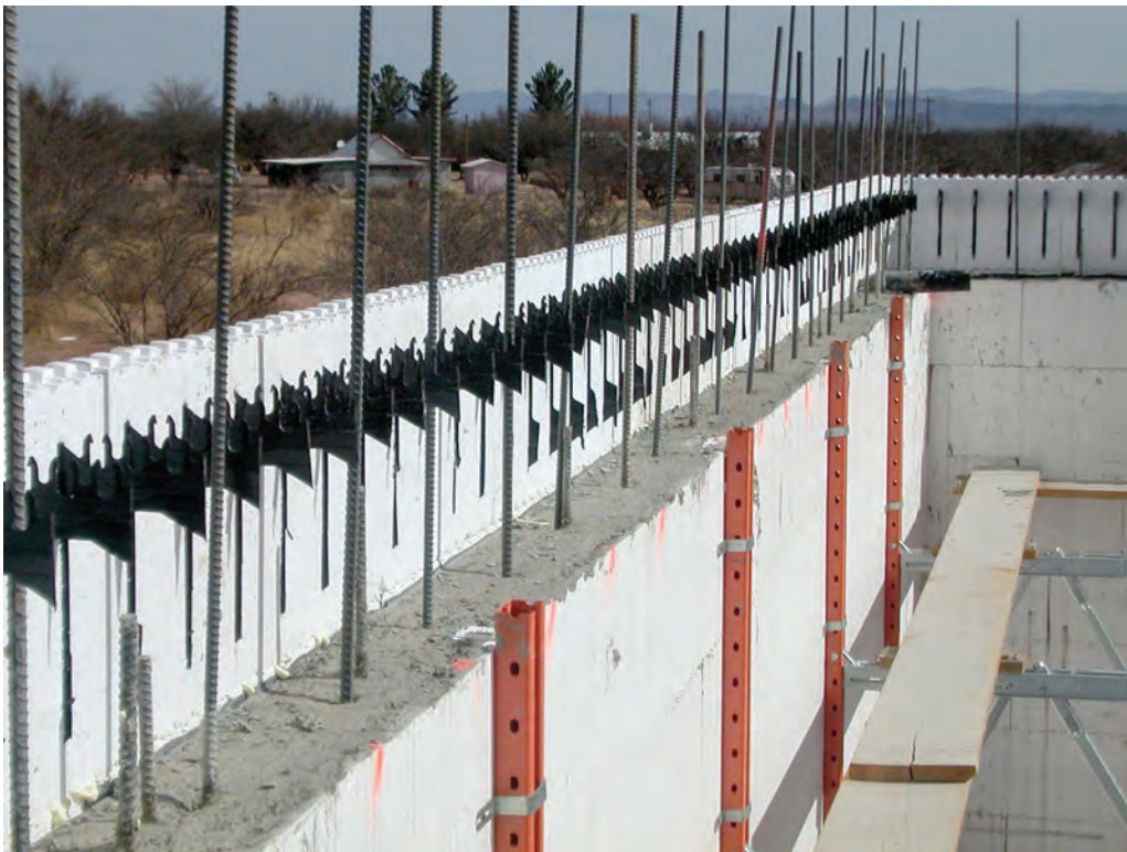
Figure 7.21 - Another view of Amvic ICF cut halfway
