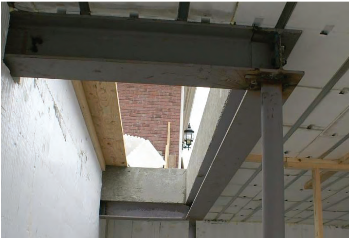
Figure 6.13 – Large sized opening in AmDeck™ supported by steel perimeter beam and column.
