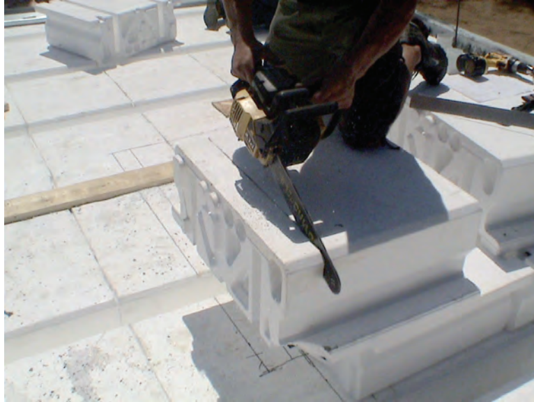
Figure 7.10 - Cutting the final block in the row
