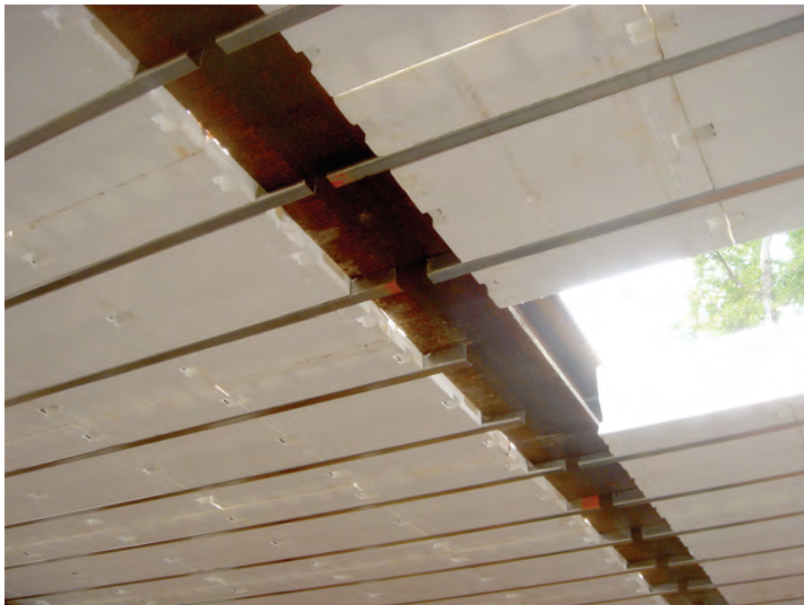
Figure 7.27 – Underside of connection between steel joists and steel beam
