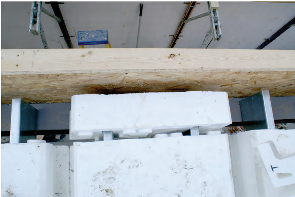
Figure 7.11 – Placement of AmDeck™ block cut transversally
