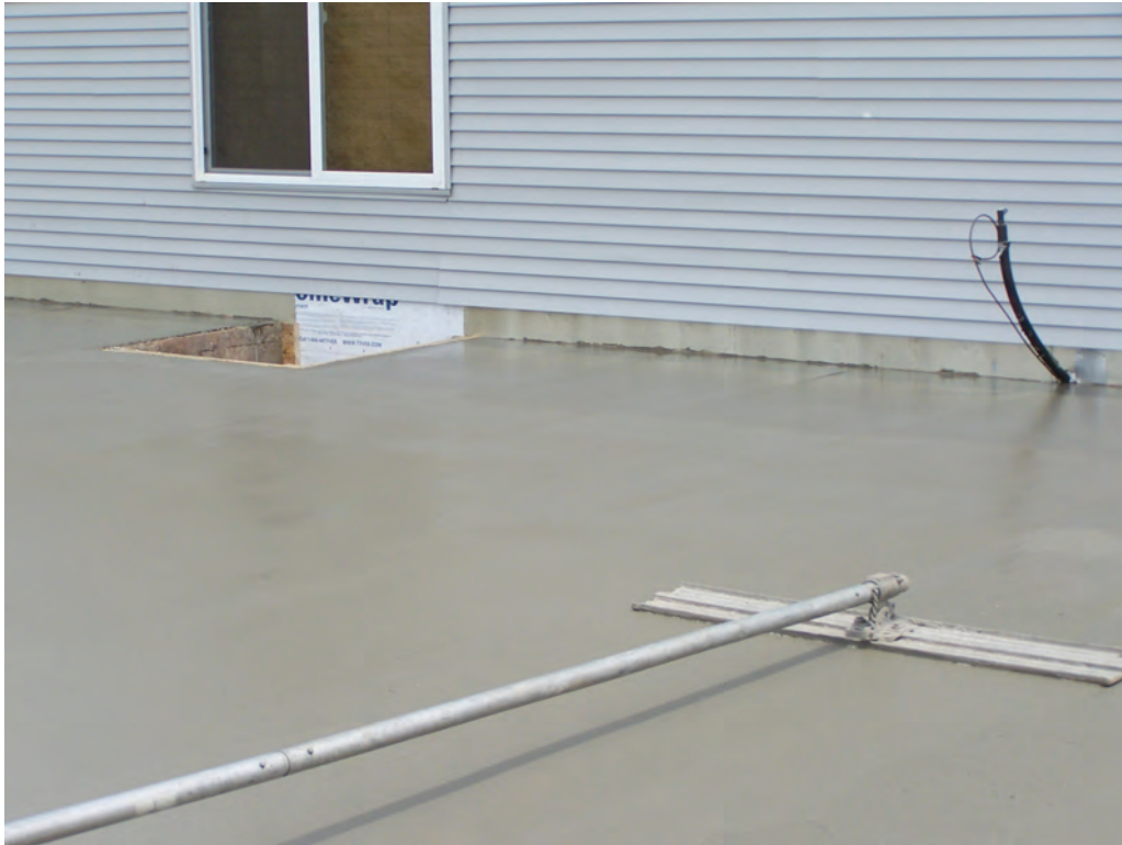
Figure 4.6 – Finishing concrete surface on AmDeck™
