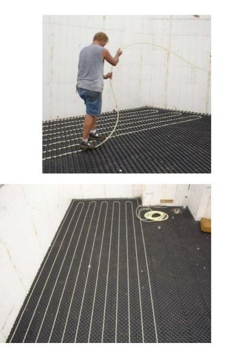
Other than ensuring the PEX is securely in the panel when making a corner, installation is as simple as walking the tube into place.
