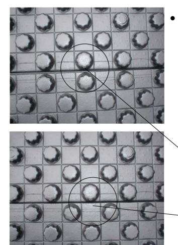
NOTE: The panels are divided into 2" squares. Each square either contains a knob or a flat and they alternate every other square. When placing the first panel of a new row you must check to verify that from row to row, this alternating sequence of knobflat-knob-flat is not interrupted. Otherwise it could cause difficulties when laying the PEX tube later on.
