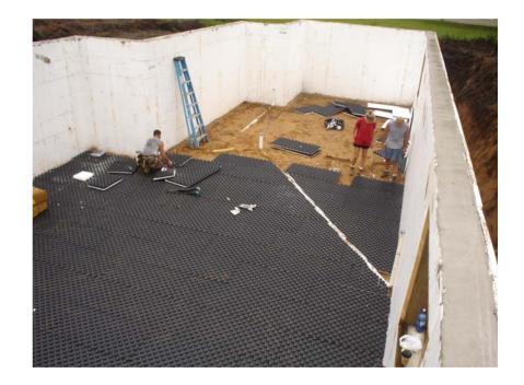
It is not required but a good idea to, after each couple of rows, walk along the interlock area of the panels to ensure that the panels are locked together.
