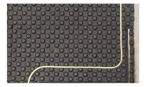
The only tip about making the PEX installation easier is that when making a turn, ensure the PEX is fully seated in the knobs before beginning or continuing a run.
