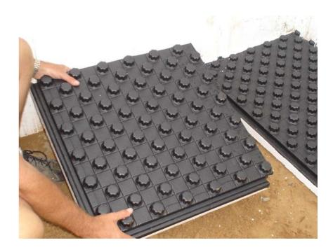
The reason for the preceding step is twofold. First, we want to make sure that we stager the joints where panels come together to avoid common seams. Second, we want to minimize waste.
