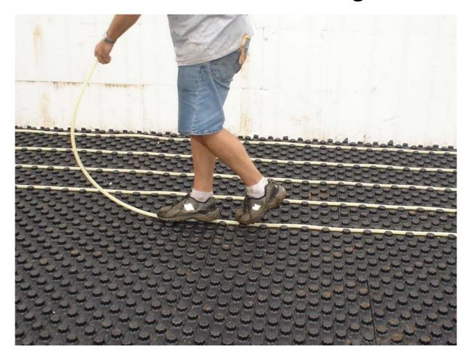
The RAZ Panel<sup>™</sup> modular board system from EZ Floor, LLC is an easily installed vapor barrier, insulation board and PEX tube holder all in one. This product allows for simple installation of hydronic radiant floor heating systems that today consist of primarily garages, basements and slab-ongrade installations where concrete is used.
