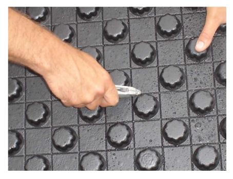
The remainder of panels that were cut in the previous step cab be used to begin the next row. If you are cutting a full panel to begin the row, the remainder will be used at the end of that row.
