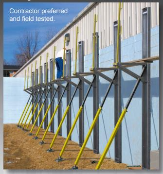
Set up and tear down takes only minutes. The brace has an adjustable built in spikeable walkway with a storable safety rail bracket required by OSHA. The walkway ledge allows for a kick-plate safety board.
